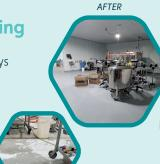
A year after installing the ComposiCoat floor finish, the floor continues to perform perfectly. There are no signs of it peeling or failing like the epoxy flooring and the ceramic surface treatment has been specified for two new plants.
