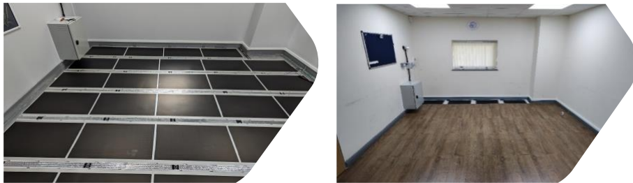
Figure 15: (Left) JustHeat Underfloor Heating Panels, (Right) Completed Demo Room at Haydale, Ammanford
